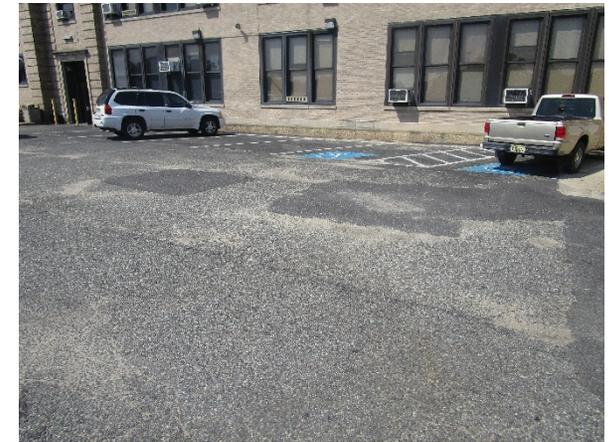
The parking spaces along the eastern side of the school can be converted into pervious pavement to allow stormwater runoff from the parking lot to infiltrate the ground. Sediment buildup is present as well as cracking and erosion. A preliminary soil assessment suggests that the soils have suitable drainage characteristics for green infrastructure.
