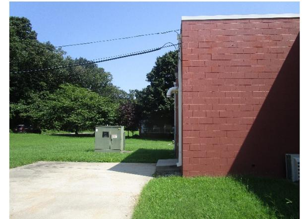
On the west side of the building, where two downspouts are present, a rain garden can be installed to capture, treat, and infiltrate stormwater runoff from the rooftop. A preliminary soil assessment suggests that the soils have suitable drainage characteristics for green infrastructure.
